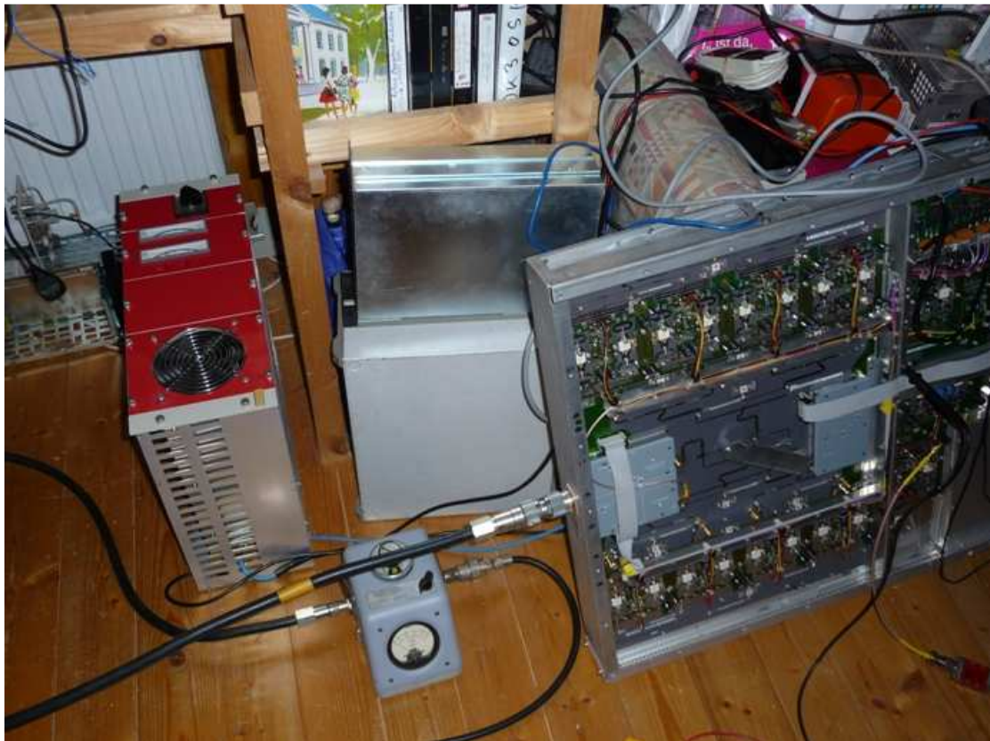
The red coloured box at the left side is a 28V power supply which should deliver about 100 amperes, unfortunately the over current protection switches off by 80 amperes, so I could not check the full output.
