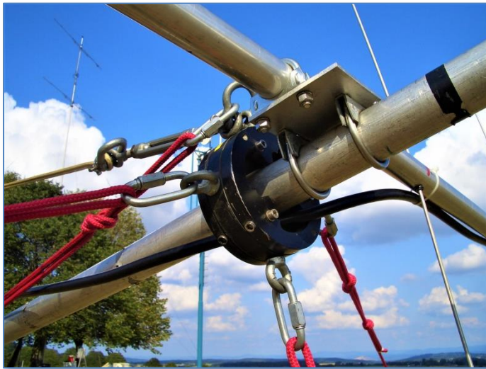
One of the pivot bearings on the antenna tower for the 2x17 elements
