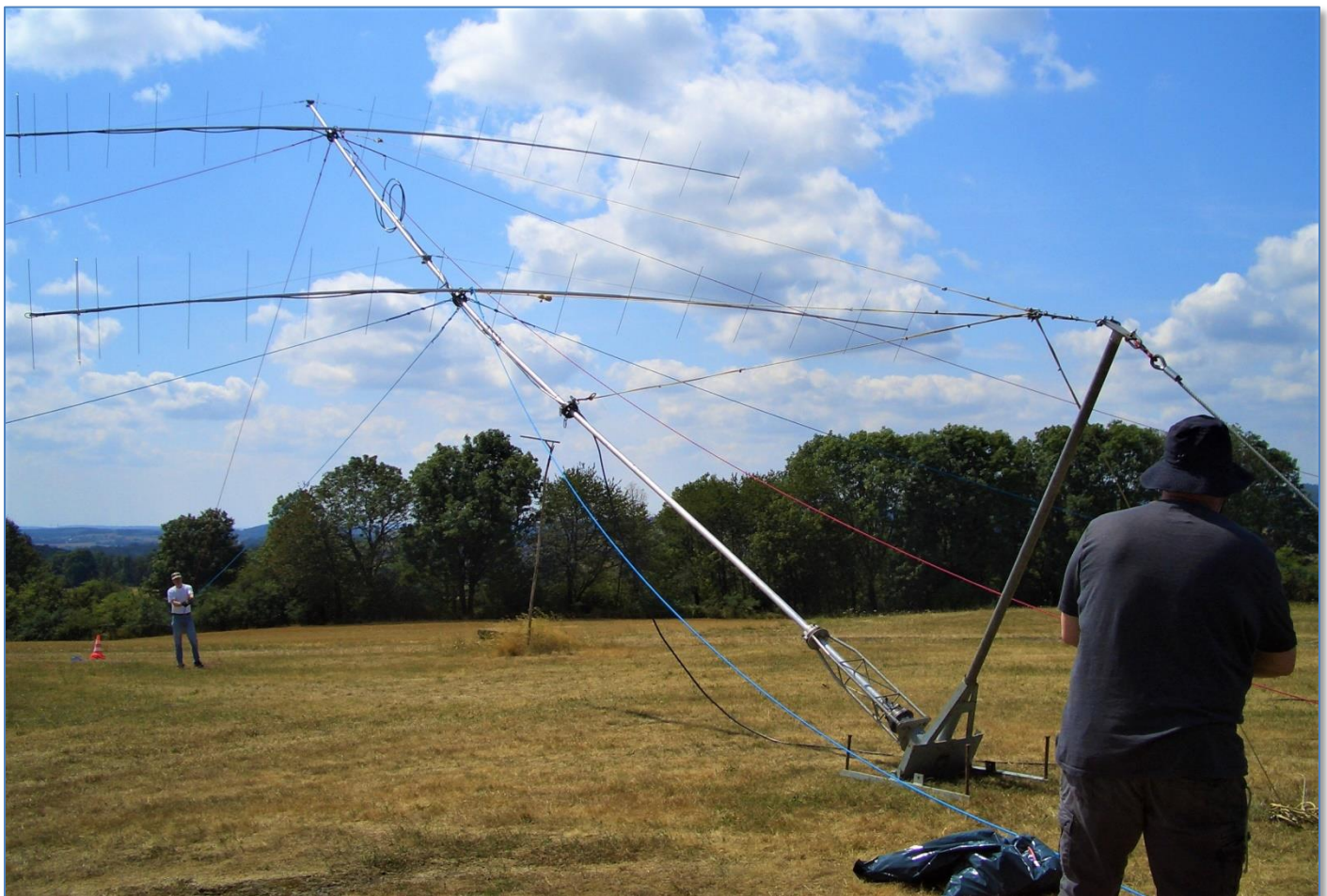
Erecting the antenna mast for the 2x17 elements Longyagis with M2
