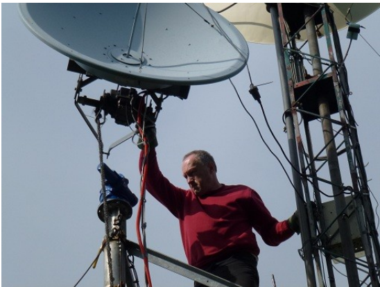
Abbildung 5: the complete 3cm system ready to lift
