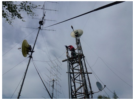
Abbildung 3: ...fixing the new rotator
