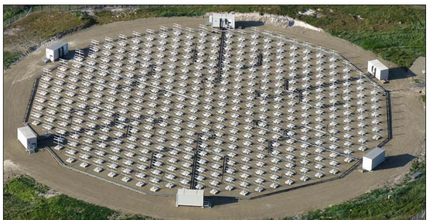
Fig. 7: The MAARSY radar at Andenes in Norway. It operates on 53.5 MHz, using an active phase-steerable array of 433 x 3-element Yagis pointed vertically. Each antenna is connected to its own transceiver, with independent phase control and a scalable output up to 2 kW. Maximum gain is 33.5 dBi, beamwidth 3.6^{\circ} and total peak transmit power reaches approximately 800 kW. The antenna field seen here is 90 m in diameter.
