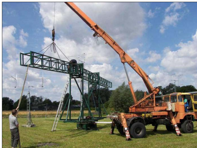
DL7APV's new tower for 70cm EME, now just the 128 Yagis are missing...
