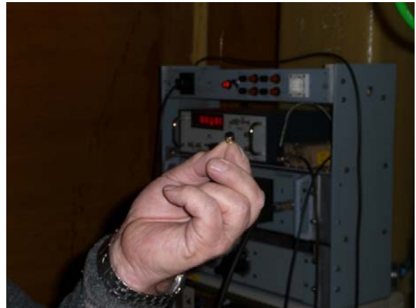
A destroyed transistor from the power supply was responsible
