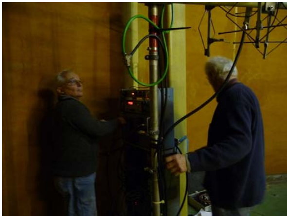
The beacon is transmitting again, DK5NI adjusts the power output
